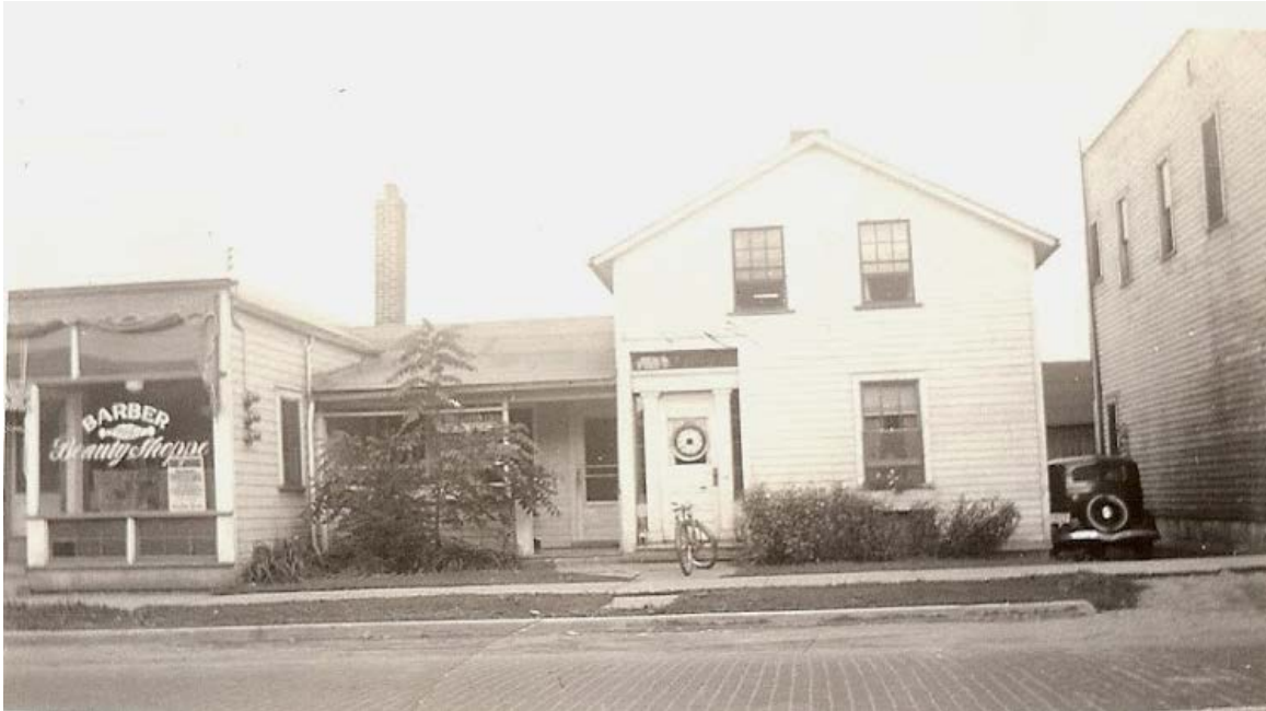
This photo from about 1937 shows the house where Carolyn Petlowany lived as a child. It was taken before the barber/beauty shop on the left became Fritz Kucklick's Radio Electric Shop. Note that Columbia Road was paved with bricks at that time.
