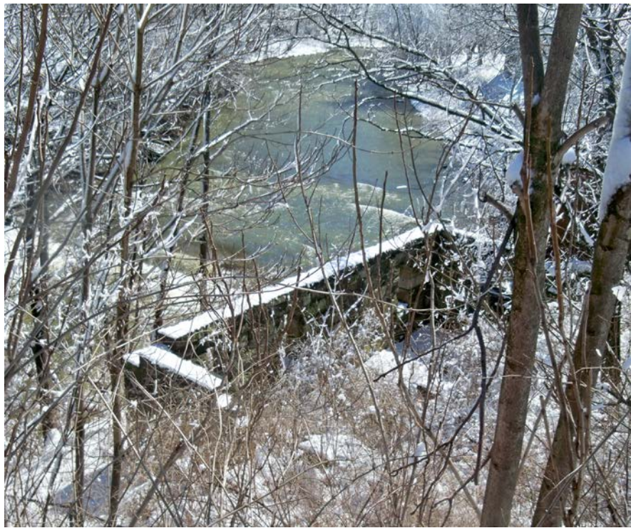
Snow frosted the stones of the foundation of Damp's Mill on Monday.
