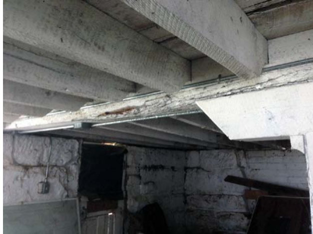
The stones and timbers of the foundation are in better condition than the rest of the barn.
