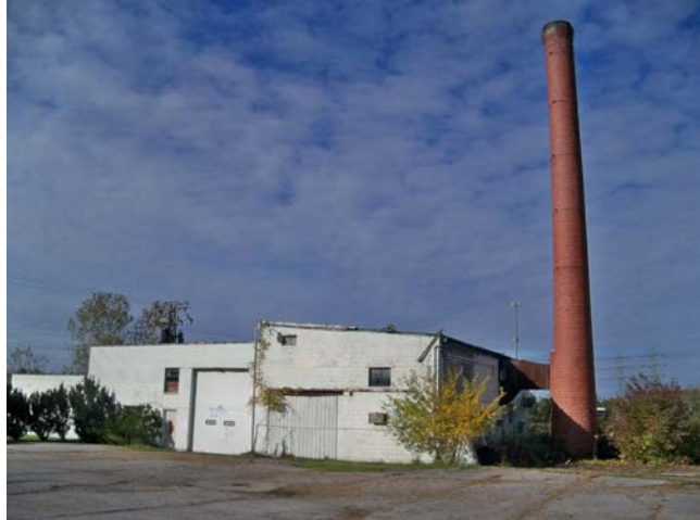
This building along McKenzie Road with a brick smokestack for its coal-fired furnace was an integral part of the Hall family's greenhouse business for several decades.
