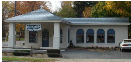
Clint Williams received an award for his conversion of the former gas station into the Olmsted Falls office of his real estate company. Photo by Bruce Banks.
