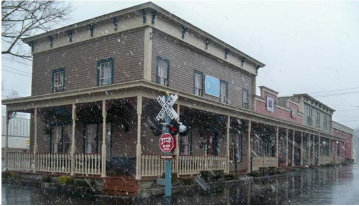
Clint Williams changed the entire character of one side of the Depositors Building.
