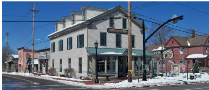
Clint Williams saw almost a complete town in the buildings he restored as Grand Pacific Junction.
