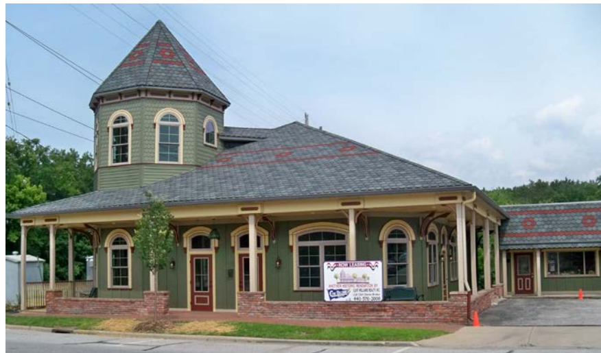
It looks like a railroad station from the late 1800s, but this is really a new store taking its place among older neighbors at Grand Pacific Junction.
