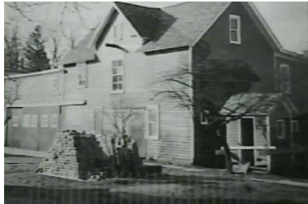
Here is the Livery Stable during the process of renovation and creation of Grand Pacific Junction. Note that the outhouse is farther from it. Photo courtesy of Clint Williams.
