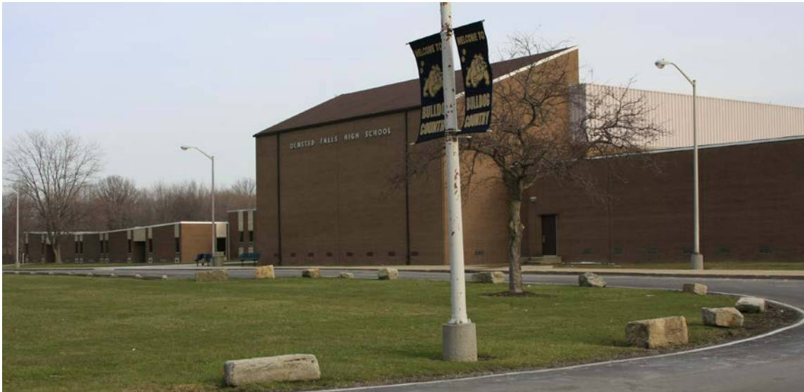
Before recent construction began to expand the high school, this is how it looked with the auditorium in the foreground.
