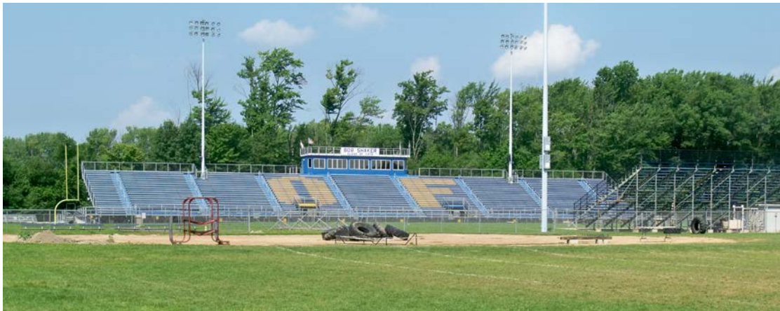
Although construction at the high school delayed the start of classes until September, Charles A. Harding Stadium was ready for the opening of football season on August 24.
